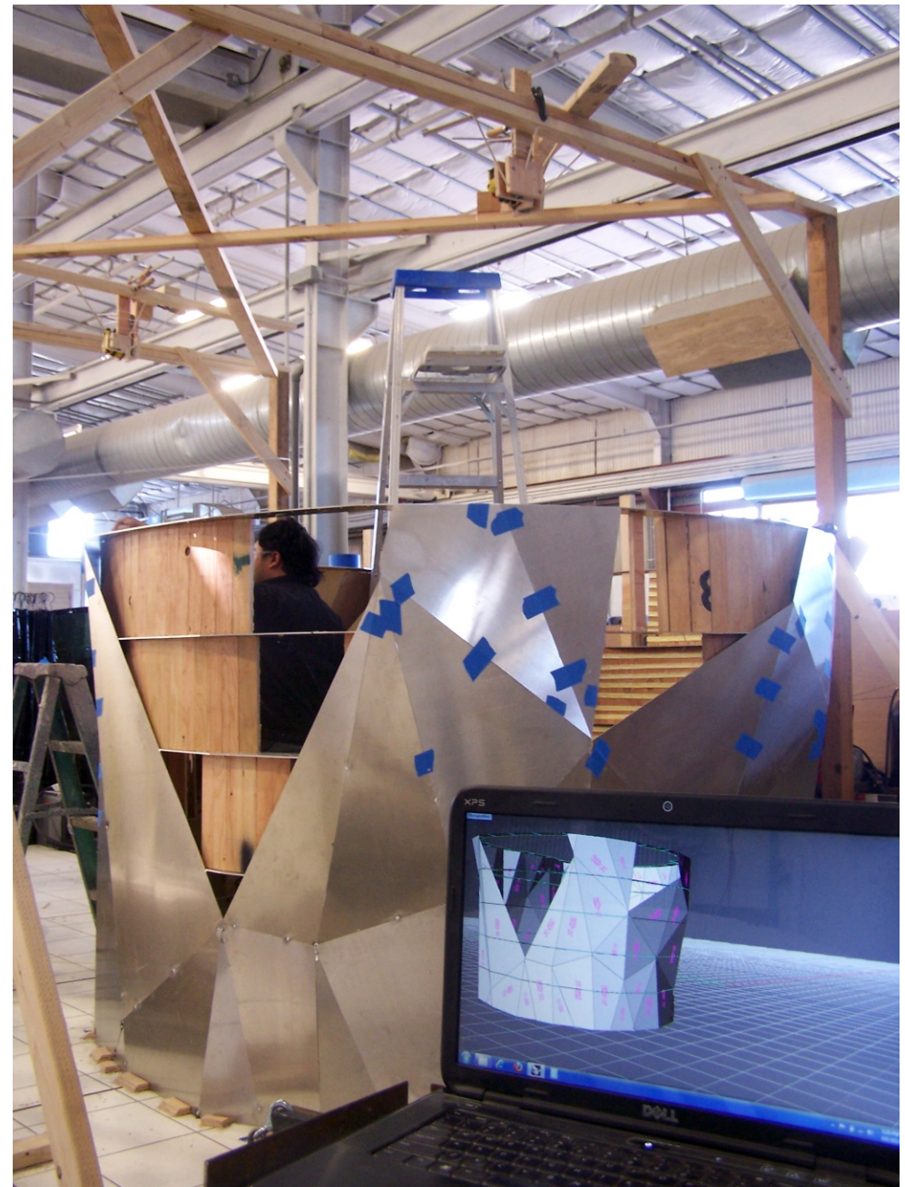
Figure 8. Assembly in various stages. The grid on the floor was supplemented with 1-foot wide, kerf-cut plywood spacers, and lasers. Once the bulkheads were in place (top-left), the inner skin panels are temporarily held in place with blue masking tape, tack welded, and set aside for final welding and finishing. Bottom-left: a graphic index of the assembly groups. The photos, from left to right correspond with groups 14, 13, and 7.
